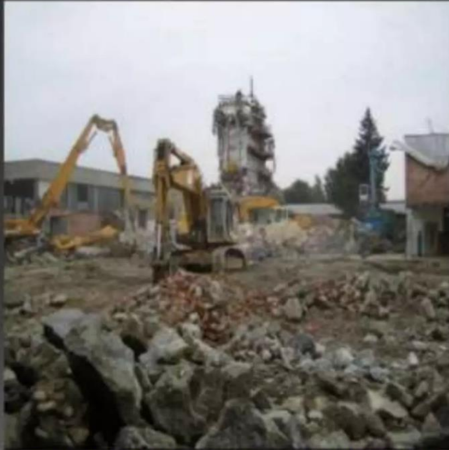
Breaking up & removing the old concrete
